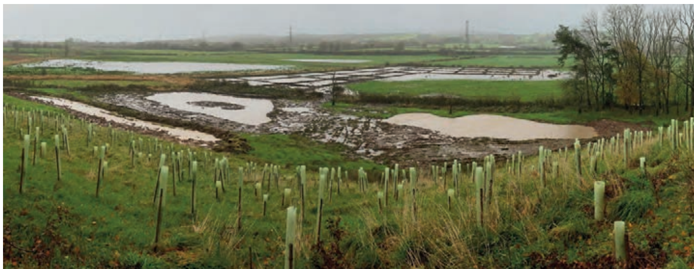
Figure 4: A panoramic view of a Wyre Natural Flood Management Project site. In the foreground is an area of woodland creation. Beyond that are two ponds created to store water from surface flows. In the background is an area of lowland peat restoration. All these interventions are helping to store water and restore critically important habitats. (©Sam Hope, Wyre Rivers Trust).
